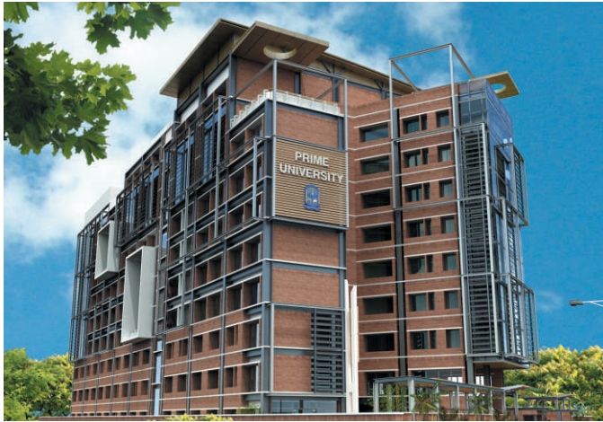
New Building of Prime University
